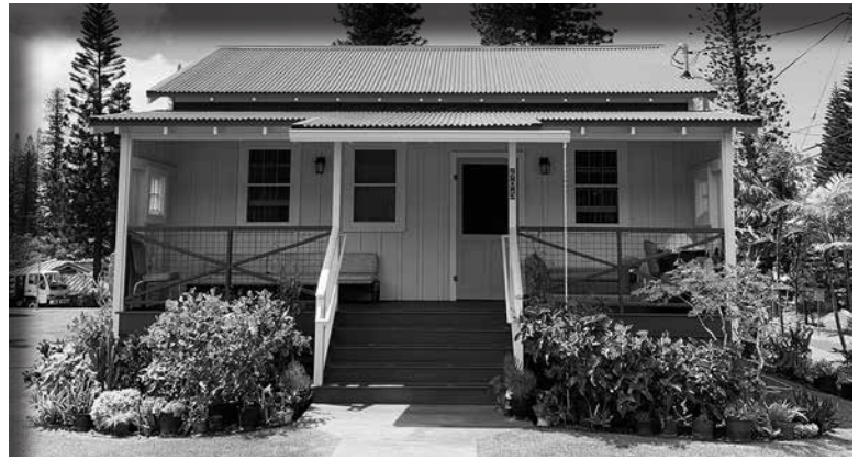
Three homes at 605 Lāna‘i Avenue were replicated to match historic features. Photograph by Historic Hawai‘i Foundation.
