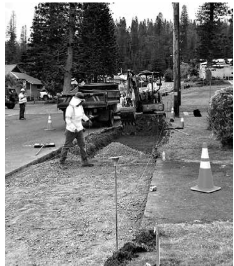
The sidewalk project in its early stage
