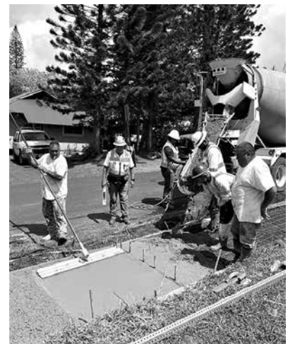
and smooths out concrete
